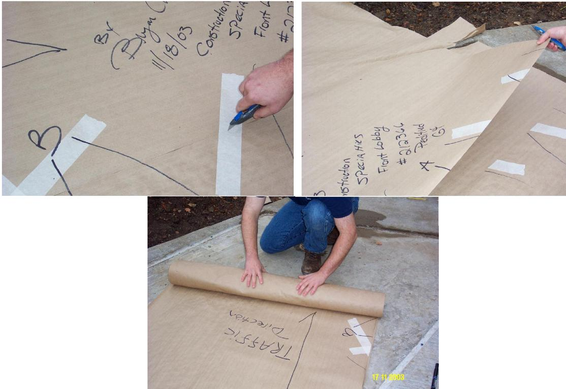
Please stack the paper so the reinforcement fibers in the paper are all running the same direction. This will prevent wrinkling from occurring. These wrinkles could alter the overall size of the template.
