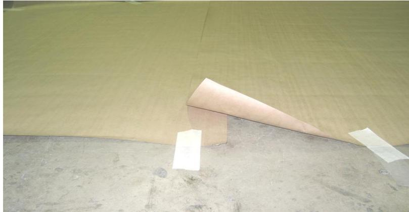
Once the paper is all laid out, place hash marks across the overlaps to aid in lining up and matching up the template pieces during assembly at the factory. This will ensure the template is assembled in the same manor at our factory as made in the field. See below. If multiple pieces of paper are used, please mark each section separately to identify the order. (ex. A, B, C, etc), if possible please include a sketch of the orientation of the sections and mark numbers.
